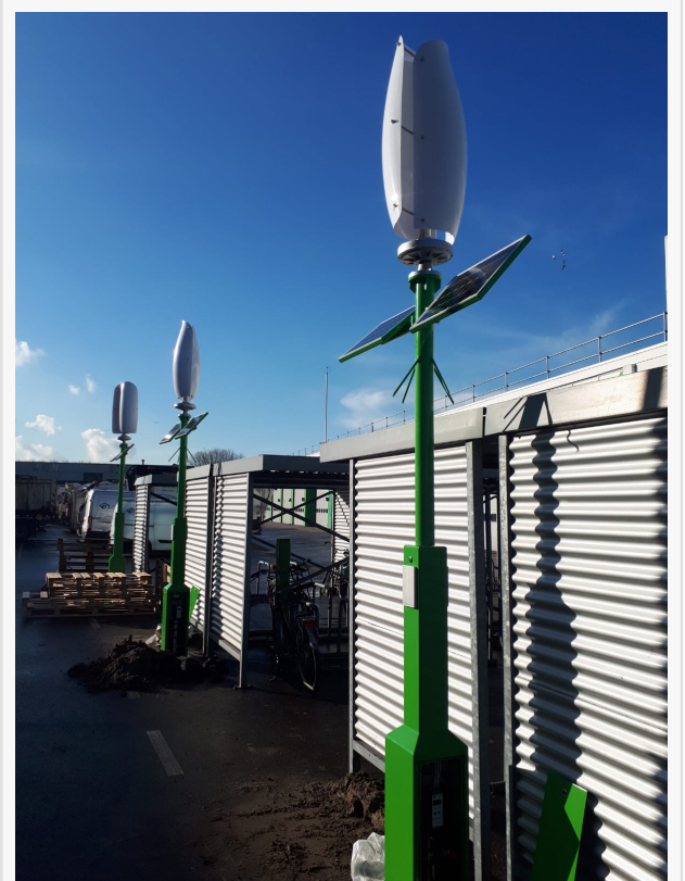
Wind and Solar E-bike Charging Poles
