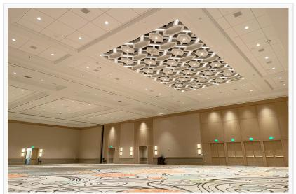
The centerpiece of the renovated Gaylord Palms Resort and Convention Center ballroom was the ceiling, highlighted by four ornate Glass Fiber Reinforced Gypsum (GFRG) fixtures totaling 3,200 square feet that were hand-assembled on-site by KENPAT. Installa
