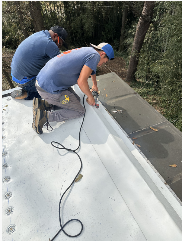
Welding IB PVC Roof
