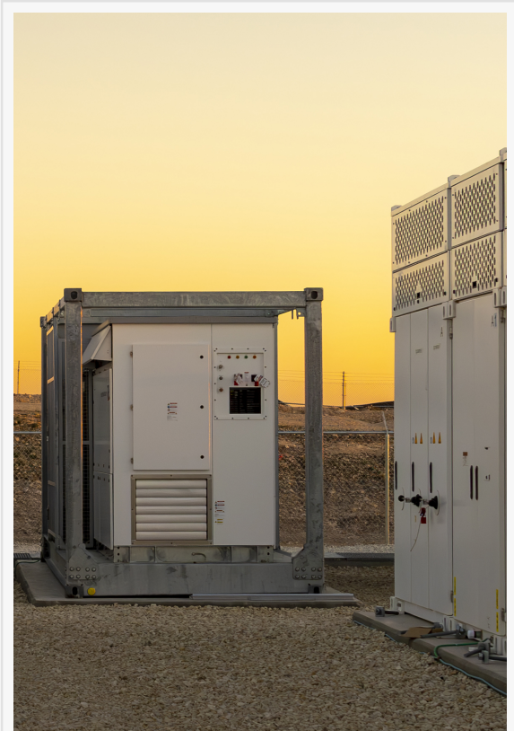
The inverter is one of the most common points of failure in an energy storage system.
