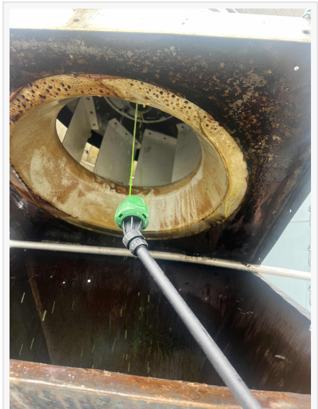
A licensed technician from Filta Kleen cleaning a exhaust duck with a power washer
