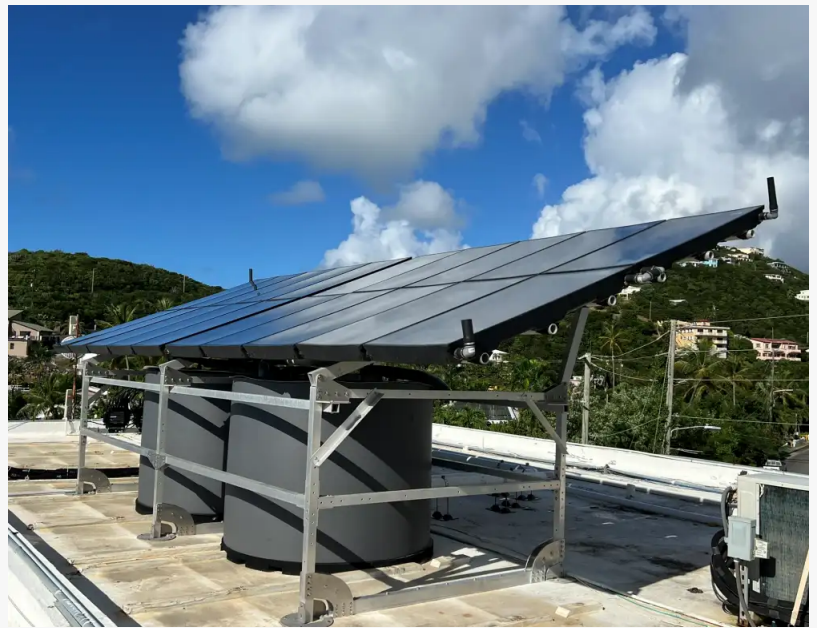
Solar thermal-electric system using PowerPanel's Thermal Storage tanks and Heat pumps at a Caribbean resort, capable of supplying the resort's entire hot water needs at a fraction of the cost of utility energy
