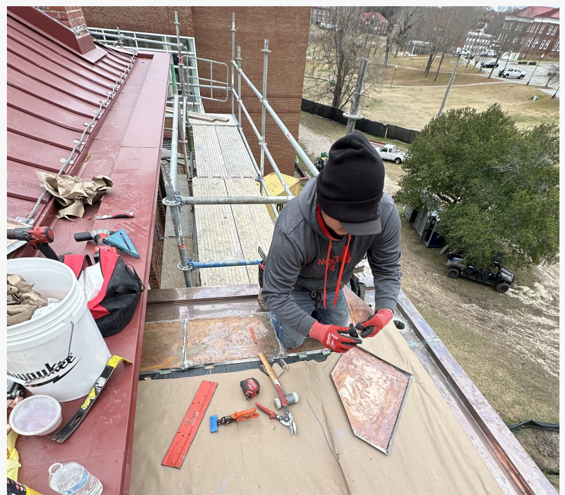
Installing Flat Lock Copper Panels
