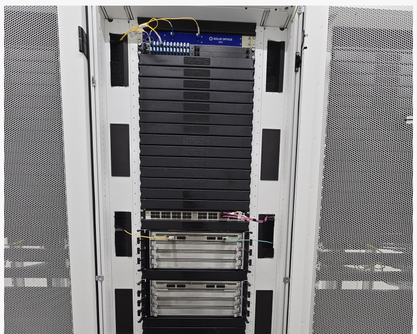
Switches fully mounted and connected in a data center rack, prepared for production use with high-speed and resilient network capabilities.
