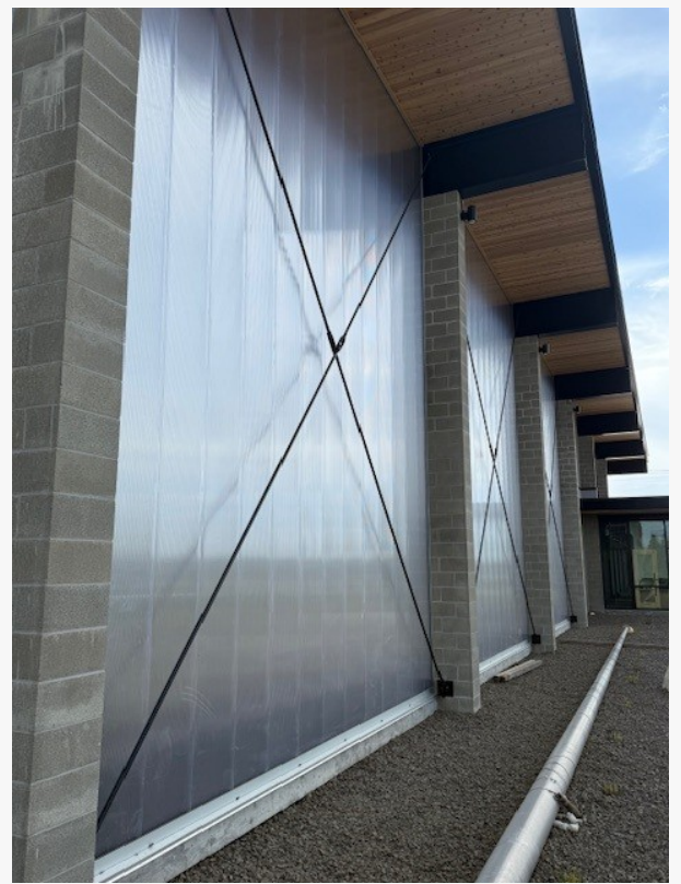
Skyview 40 is a 40MM transparent polycarbonate encapsulated into an aluminum framing system.
