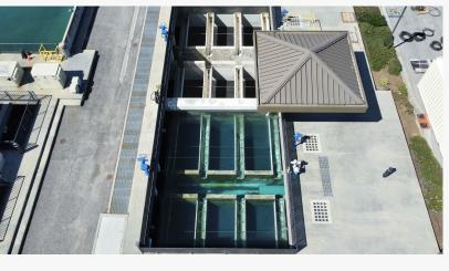
a 10-inch layer of sand and 4 feet of fresh GAC media, designed to optimize filtration efficiency and water quality. A major highlight of the project was the installation of approximately 32,000 new underdrain nozzles and 12 new actuators, stands, valves, and deflectors, which are essential to the plant's filtration and backwash operations.
