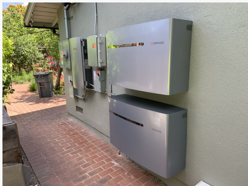
Simmitri Inc. Solar Battery Installation
