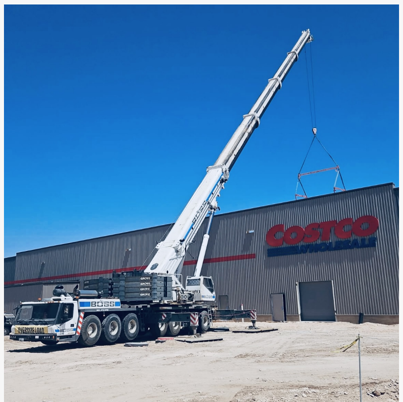
BOSS Crane & Rigging's Grove GMK7550 lifting 26,000 lb. air conditioning unit at a Midland, Texas Costco location.
