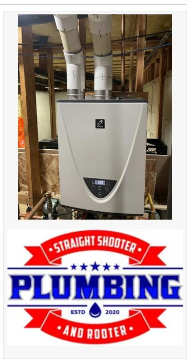
Lower Energy Bills and Increased Savings Tankless water heaters can improve both efficiency and utility cost management. By heating water only when needed, these systems can reduce standby energy losses associated with conventional storage water heaters. The compact design also frees up physical space, making it a practical solution for homeowners with limited utility room capacity.
