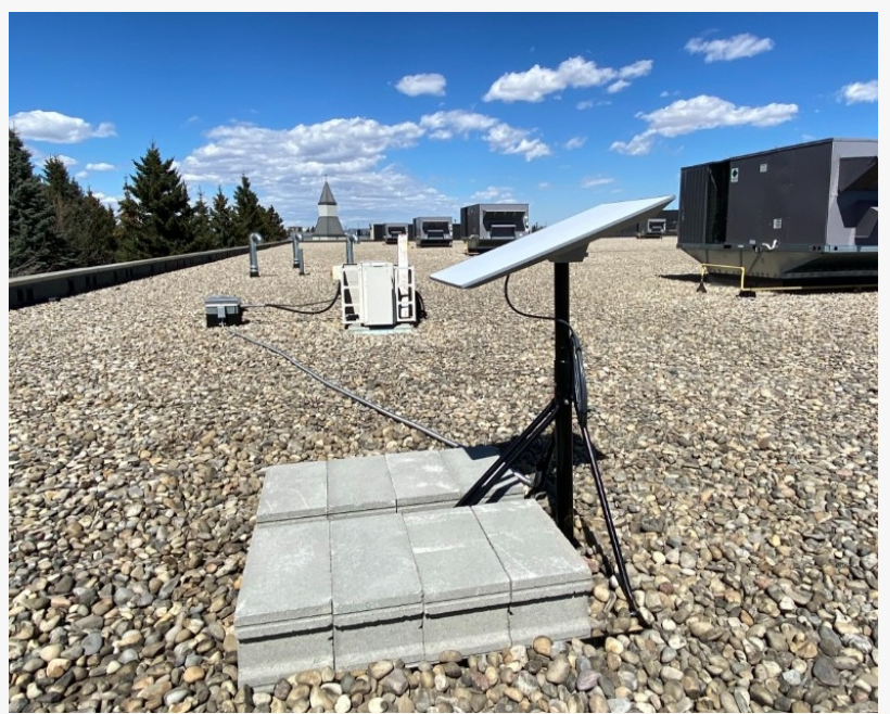
Professional Starlink Installation Georgia
