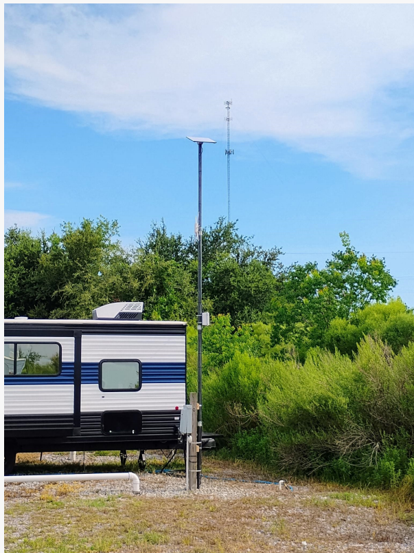
Professional Starlink installation Colorado
