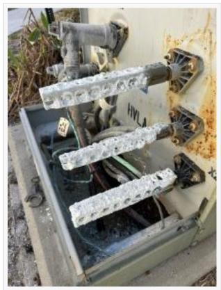
Crews replaced this pad-mount transformer's corroded secondary bars with new submersible secondary bars and correctly labeled all equipment.
