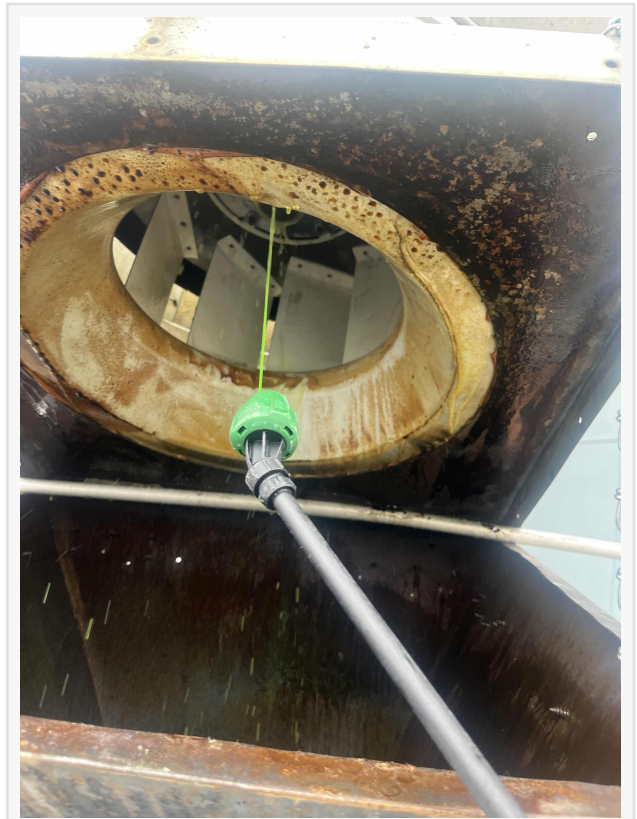
A licensed technician from Filta Kleen cleaning a exhaust duct with a power washer
