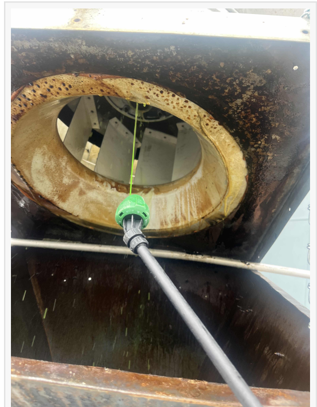
A licensed technician from Filta Kleen cleaning an exhaust duct with a power washer
