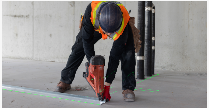
Installing Tracks with the XR Projector's Laser Projection
