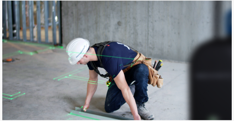
Laser Projection for Floor and Ceiling Layout with the XR Projector by Mechasys
