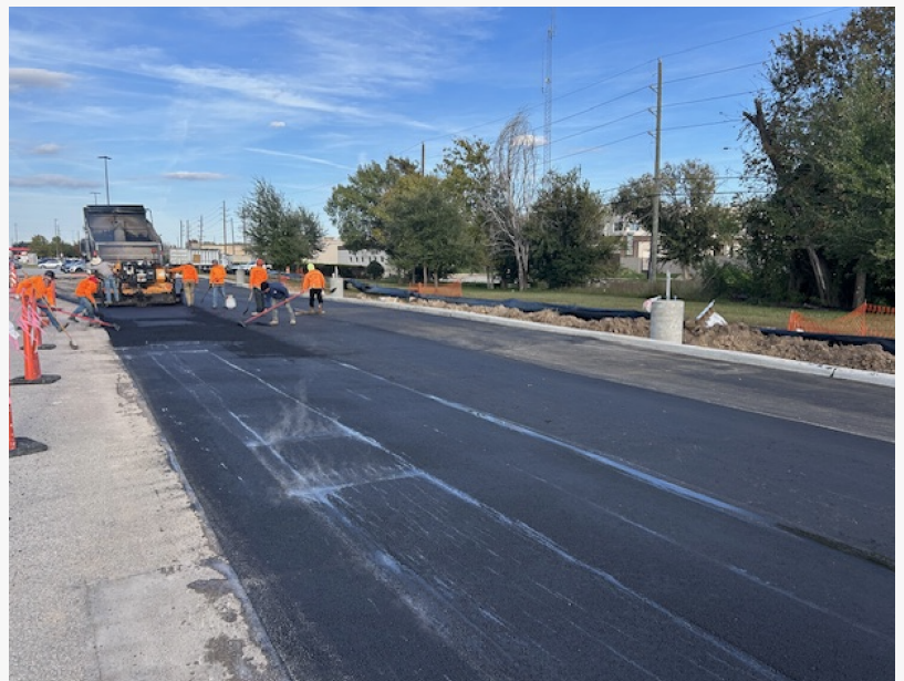
Team working hard on Asphalt Overlay
