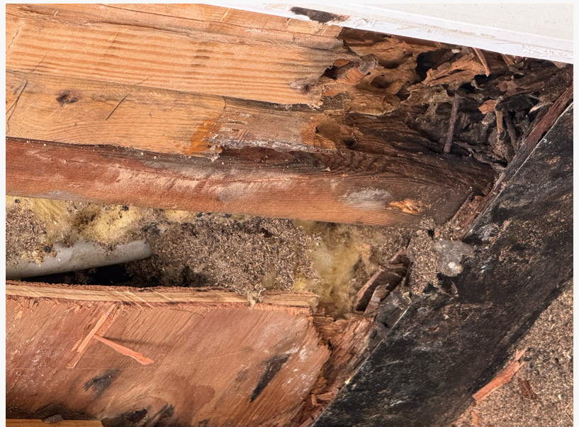
Carpenter Ant Damage
