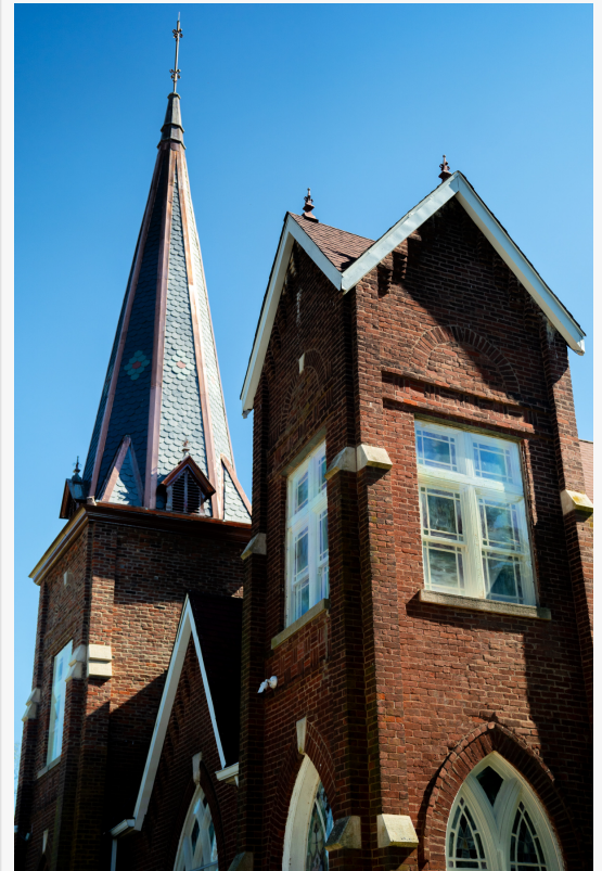
The natural slate on the steeple spire was meticulously installed to mimic the original design on the steeple built in 1900
