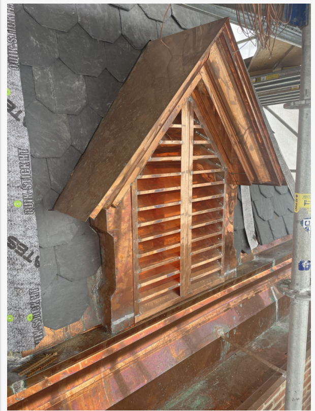
Custom copper dormers were recreated during the complete restoration of the steeple on the 1900 structure built on the birthplace of Jefferson Davis.
