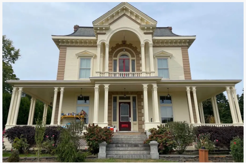
Exterior Painting in Franklin County
