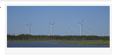
The Lamèque Wind Farm has been operating for nearly 15 years, since March 2011. The site features 30 Acciona Windpower turbines and has a rated production capacity of 45 MW, enough power for more than 8,000 New Brunswick homes.
