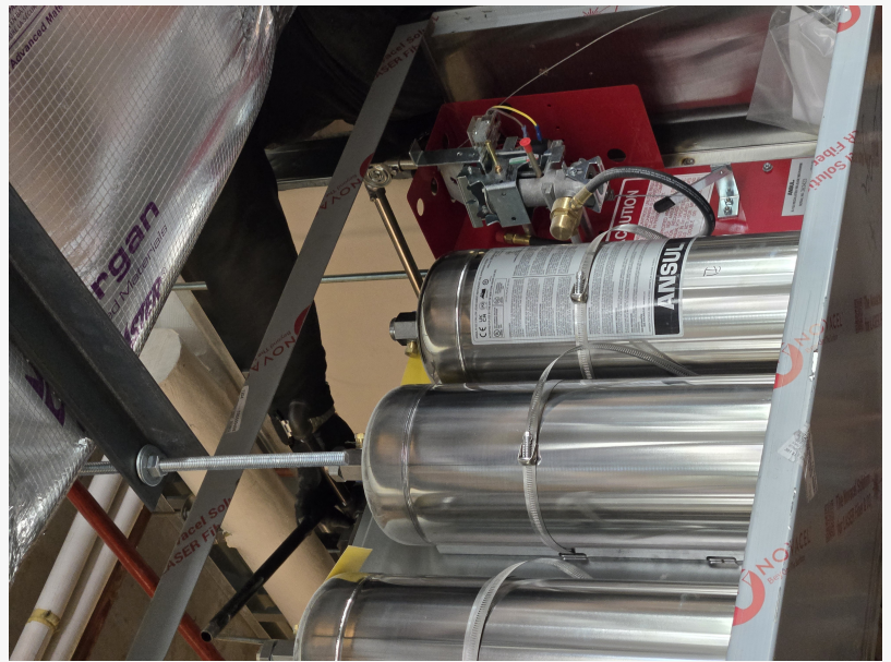
A Ansul Fire Suppression System installed in a restaurant that Done Right Hood and Fire Safety Services Located in South Florida
