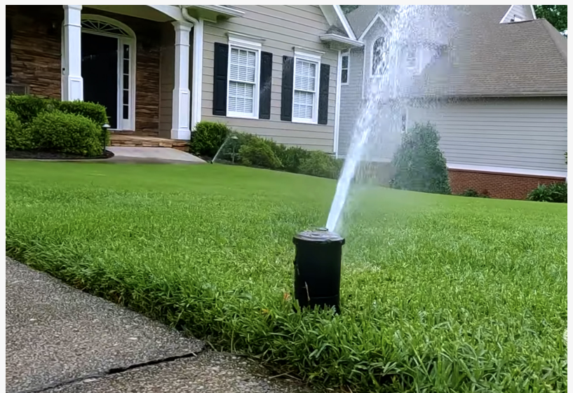
Pop-up irrigation rotors are typically used to irrigate larger areas of the yard.
