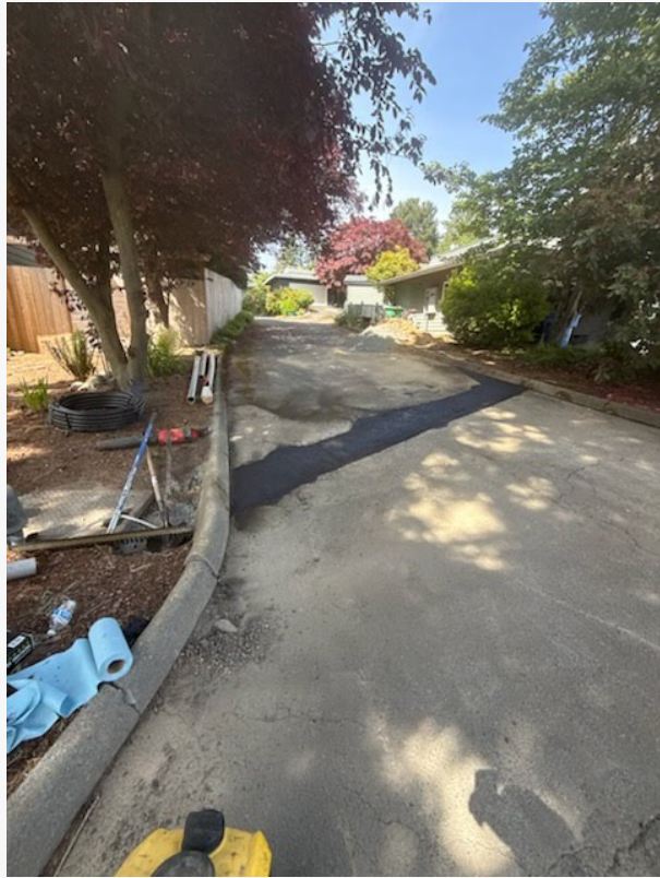
Indepth Excavation fills and covers the trenches with asphalt
