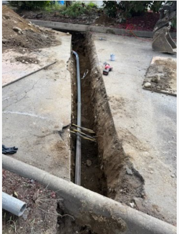
Complete Saw Cutting of the Main Road for the Excavation Project with Indepth Excavation
