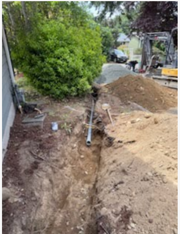
Using the mini excavator to dig out around the home for the electrical line
