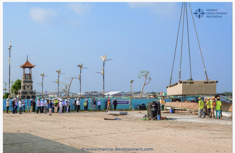
A defining moment at the Bali Benoa Marina site as the first concrete pontoon is lifted for installation, witnessed by project teams, engineers, and key stakeholders
