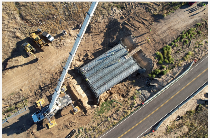
Adams County Bridge - Deck Installation
