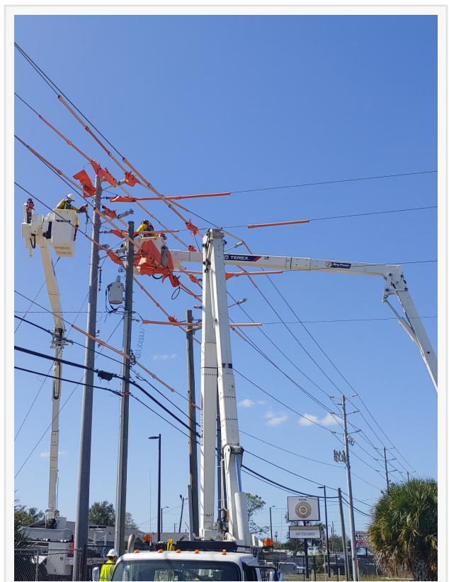
Crews framing a new pole with side-by-side feeders from the existing pole with stacked circuits.
