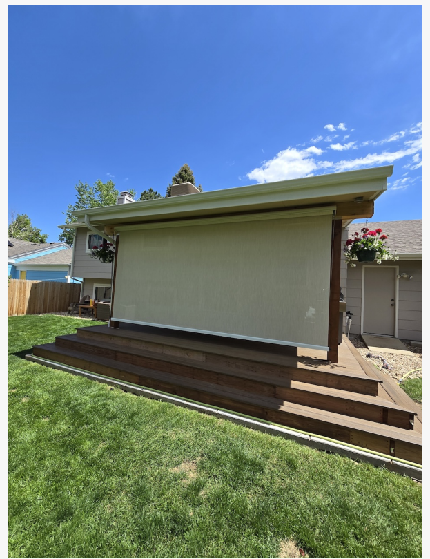
Outdoor Shade Installation in Louisville
