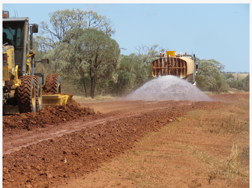
RST Solutions products added to water trucks to stabilise road access to mining companies' sites
