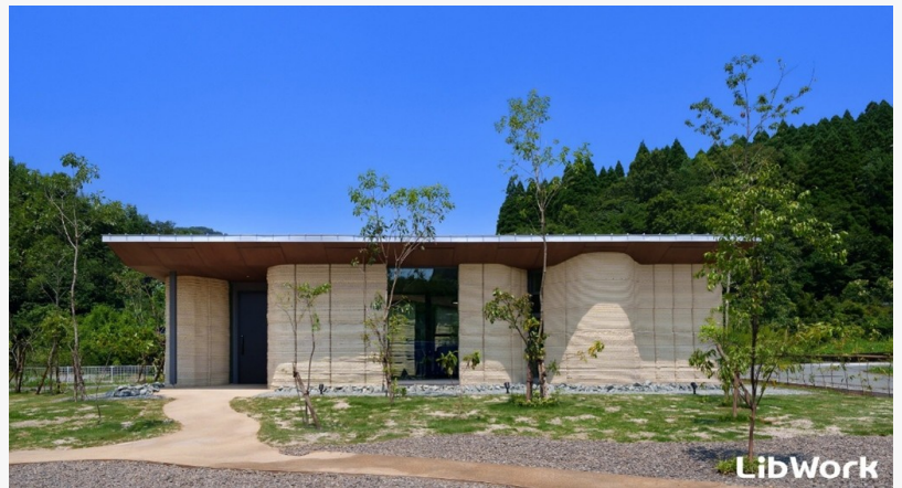
Exterior of Lib Earth House Model B
