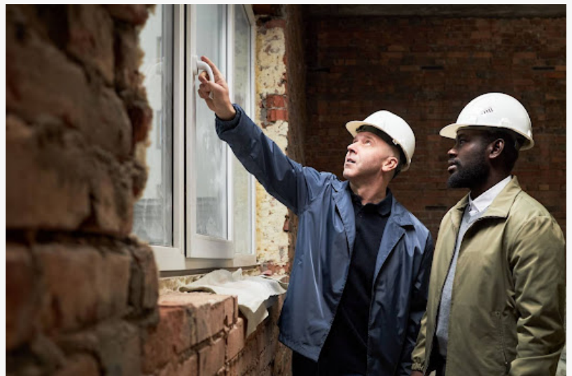
Two restoration professionals conduct damage assessment on-site after storm impact.
