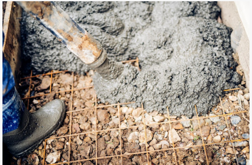
Close-up of a cement pump hose pouring durable concrete mix at a building site.
