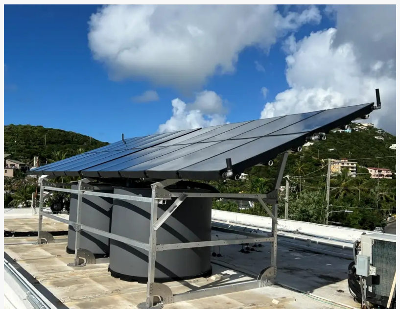
Thermal Energy 2 tanks with PVT and Heat Pump
