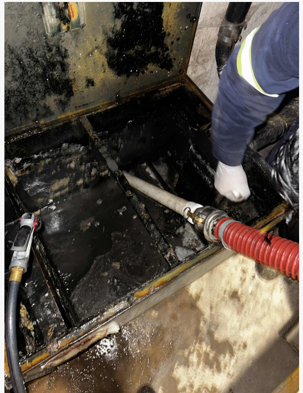
Green Oil Recycling Suctioning the Grease out of a Grease Trap at The World Trade Center
