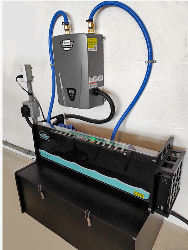
HUG Hydronics system paired with an electric boiler
