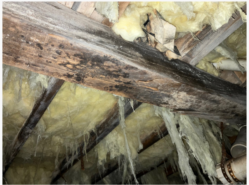
Moisture Damage / Fungi under a home
