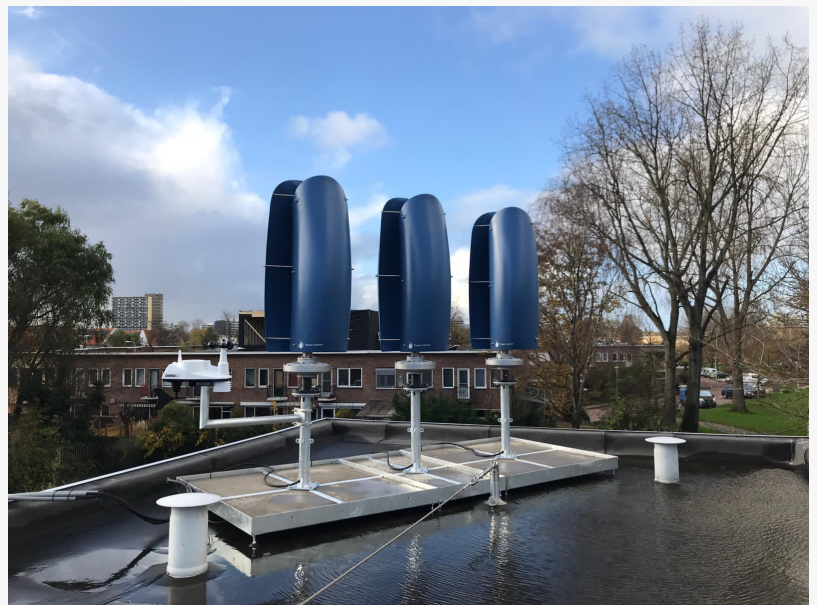
Three installed small size Wind Tulips
