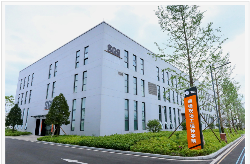
SGS's Renewable and Advanced Energy Laboratory at Chongqing, China
