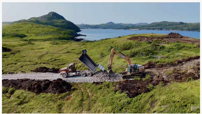
Atlantic Spaceport Complex - Construction
