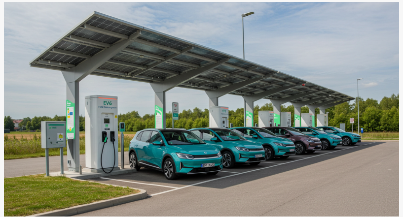
Off grid electric vehicle charging stations built with carports and backup battery power
