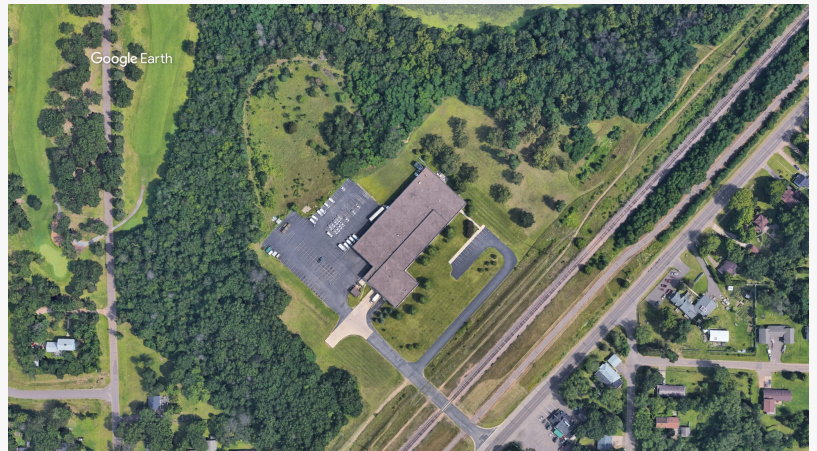
Aerial view of Atlas Manufacturing's new 48,000 sq. ft. facility in Lake Hallie, Wisconsin. The expansion consolidates operations and enables future growth.
