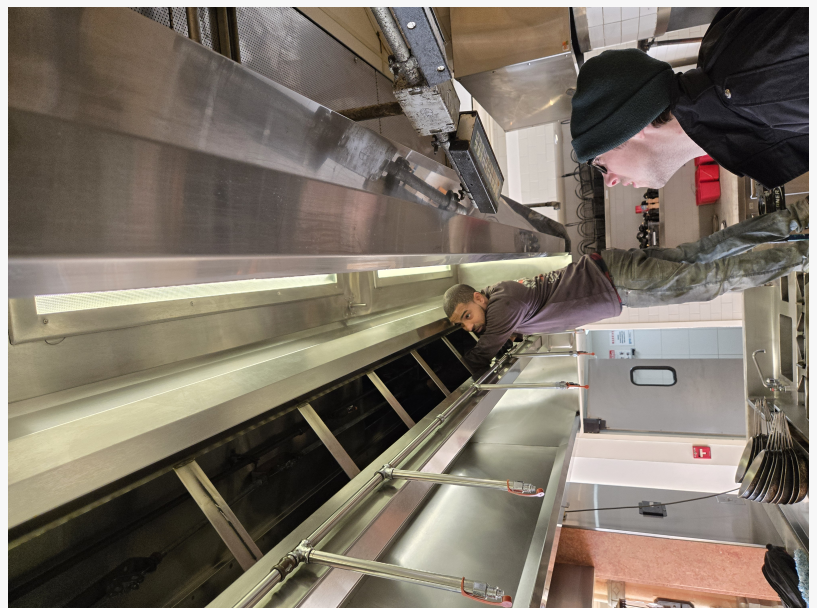
A done right hood and fire safety technician installing a fire suppression system at a local restaurant.
