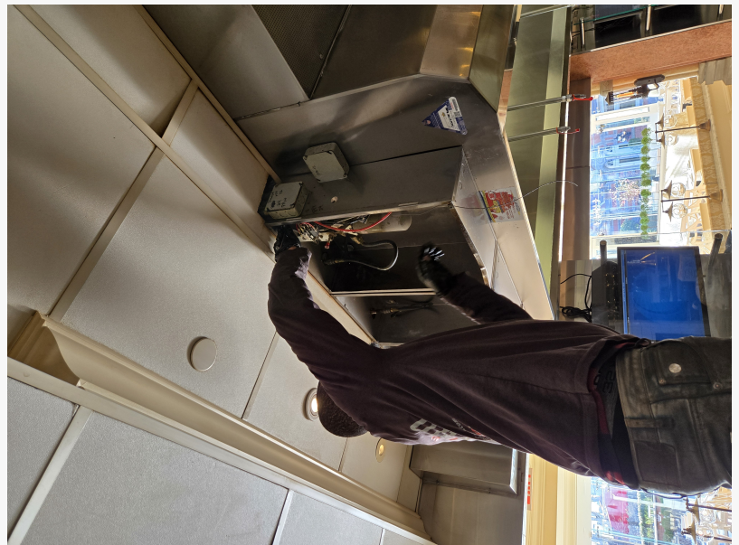
A done right hood and fire safety technician installing a fire suppression system.
