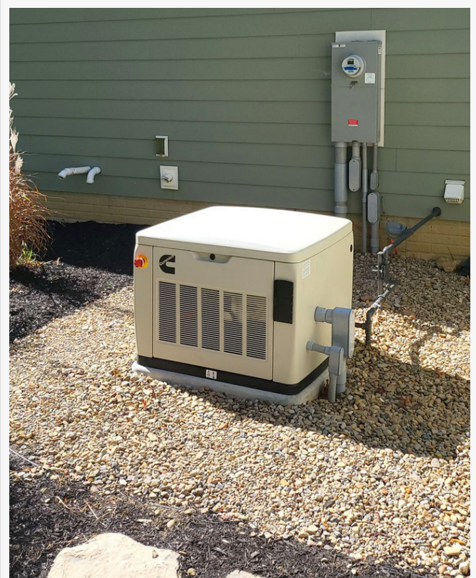
Cummins RS20A air-cooled generator installation - offers managed whole house coverage for many homes up to 3000 sq ft.
