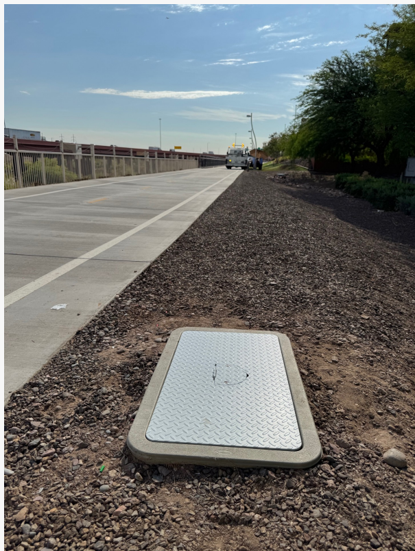
Completed Installation of In ground J Box in Tempe, Arizona
