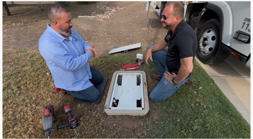
In Ground J Box Installation in the City of Tempe, Arizona
