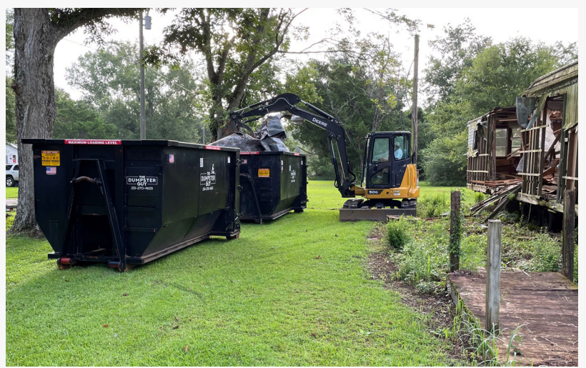
Mobile Home Demolition & Removal Baldwin County AL
