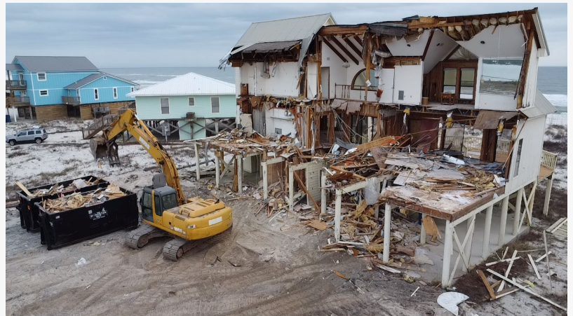
House Demolition Baldwin County AL
