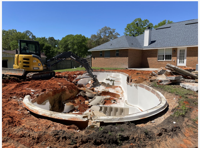
Pool Demolition Baldwin County AL
