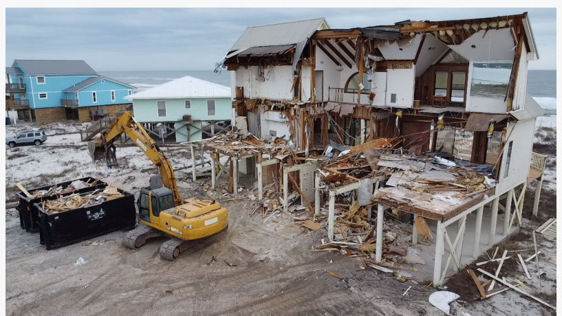
House Demolition Montgomery AL
