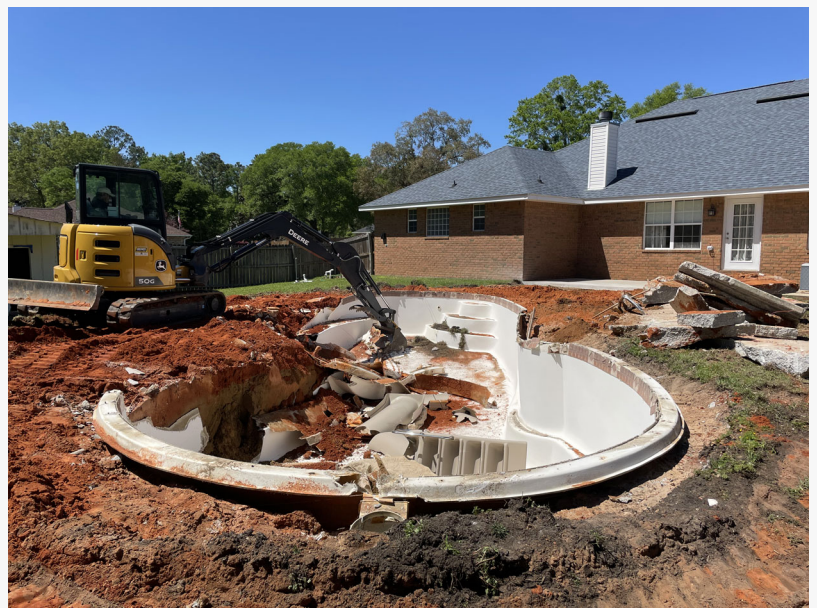
Pool Demolition Montgomery AL
