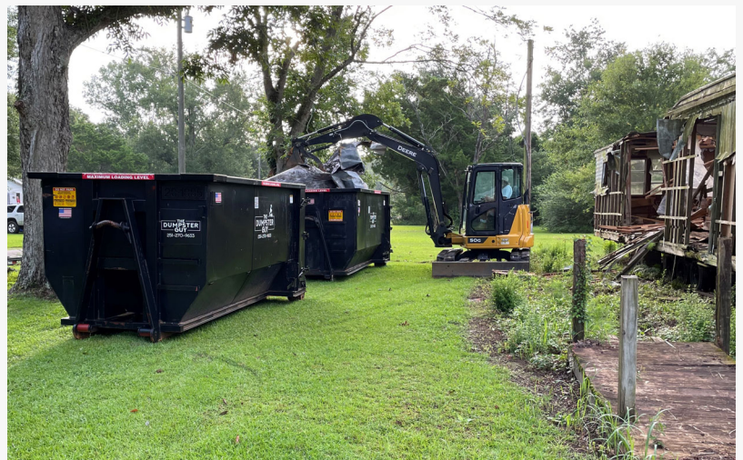
Mobile Home Demolition & Removal Montgomery AL
