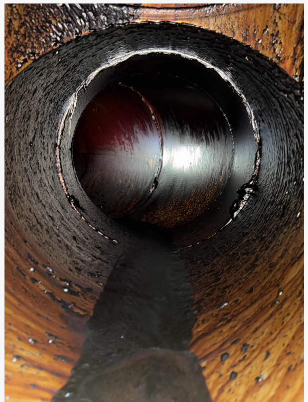
A dirty exhaust duct that is about to be cleaned by a Filta Kleen technician
